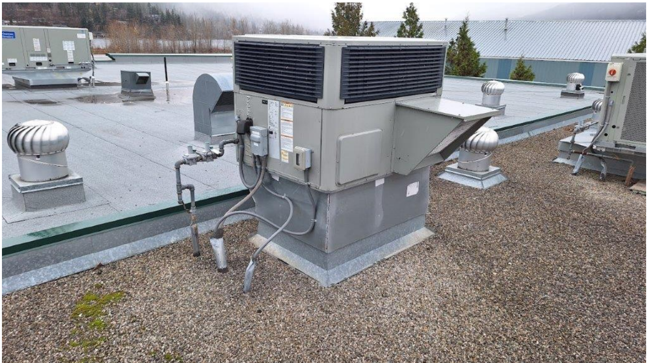
Rooftop unit typical penetration detail
