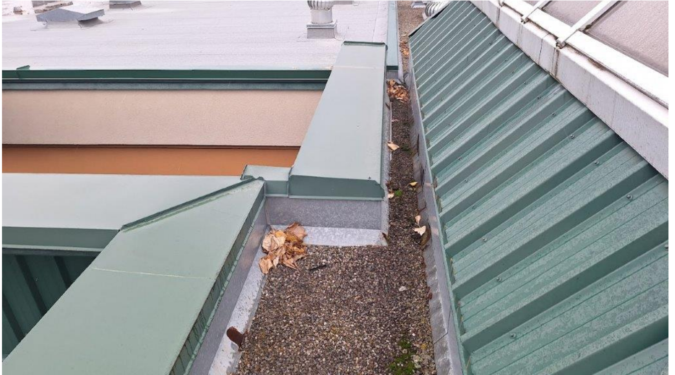
Transition between new roof and old roof above lobby – facing east
