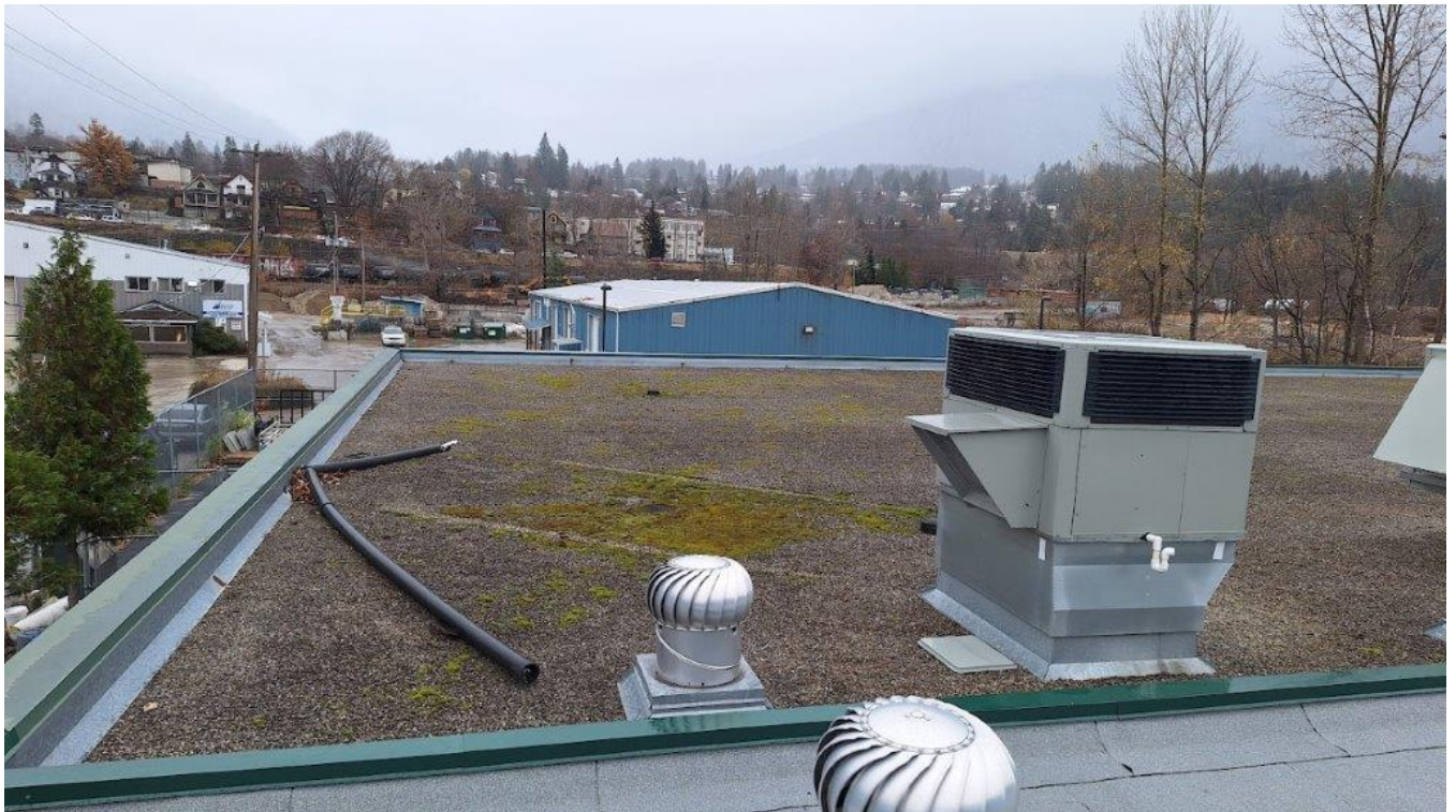
Old roof – facing south
