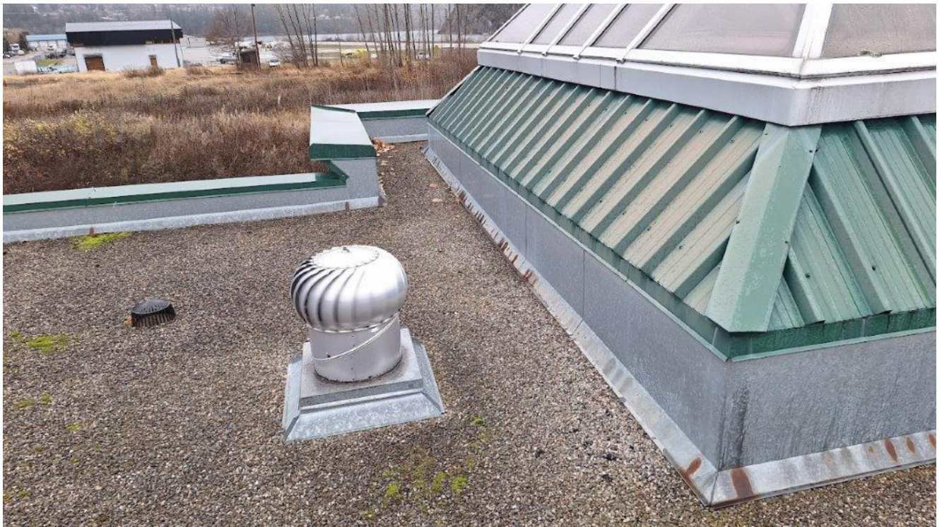
Old roof above lobby – facing west
