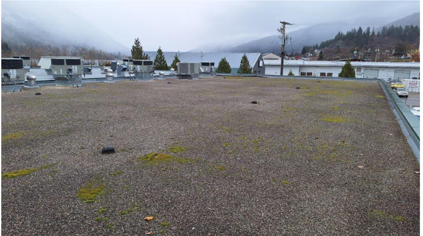
Old roof – facing east from SW corner
